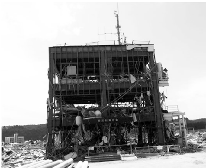
Fig. 1 The Disaster Prevention Center in Minamisanriku, after earthquake and tsunami in March 2011. Photo U Hiroi 2011
