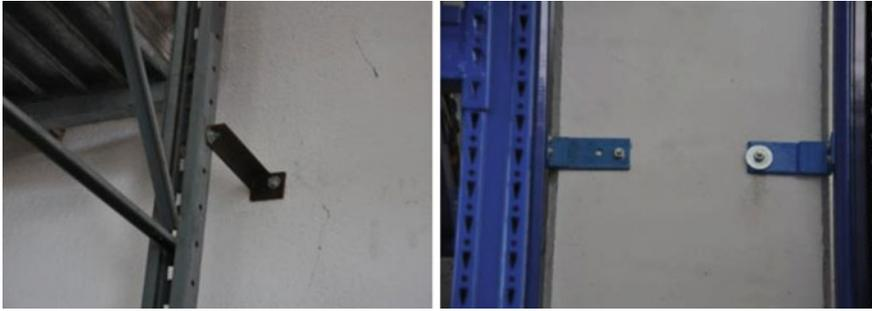
**Fig. A. 3** Detail of anchored rack
