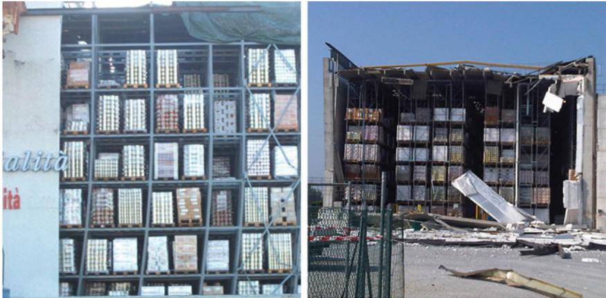
**Fig. A. 6** Onset of global collapse mechanism
