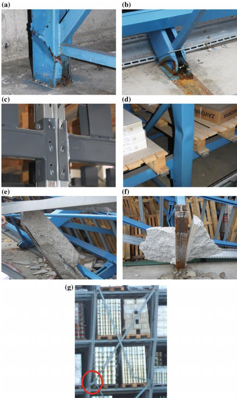
**Fig. A. 2** Critical issues observed on **a, b** base connection, **c** beam-to-upright connections, **d** upright, **e, f** base support, **g** bracing system
