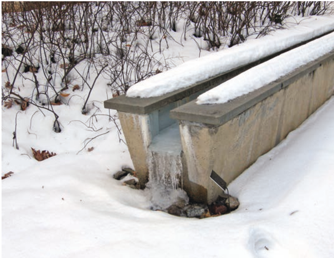
Figure 5.1. Frozen rain suspended from runnels at the Swarthmore Science Center makes people recognize the significance of rain even in winter (design: ML Baird & Co., Einhorn Yaffee Prescott; photograph: Mara Lee Baird).
