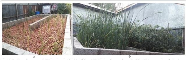
Fig. 2 The pilot scale two-stage HSSFCWs planted with *C. alternifolius* and *T. latifolia* at the start of operation (**a**) and fully grown plants during the experimentation (**b**)
