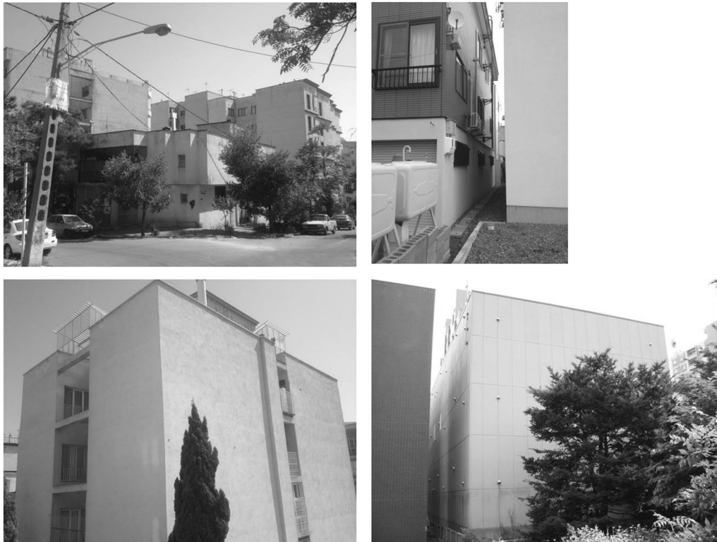
Fig. 2 (Top Left) Inner courtyards as mere light shafts in housing blocks in Iran, whereas in the Japanese case (Top Right) open spaces are shaped as side setbacks. There is a hypothesis that redistributing the open spaces in Iranian case and introduce wider inner courtyards will contribute to the better ventilation and perception of these open spaces in residential blocks (Bottom). Facades with windows are colored in grey. (Left) Hayat-khalvats as light shafts in housing blocks in Shiraz. (Right). Side setbacks in Sapporo case
