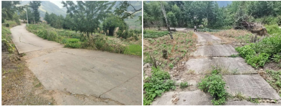
Fig. 5 Road cracking at the landslide body in Lianyun Village
