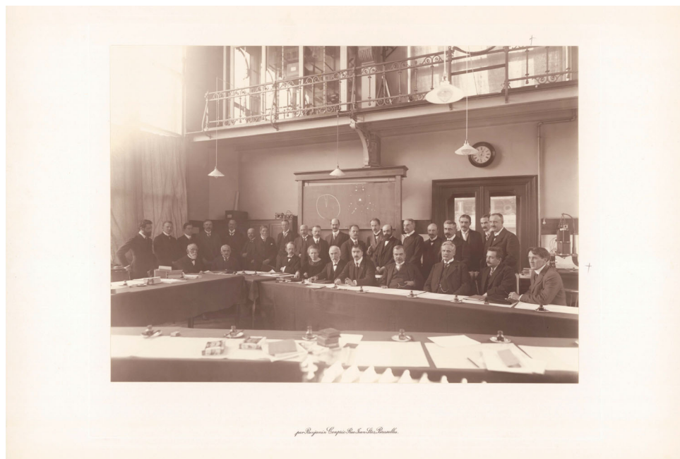
This is a less-known “indoor photo” of Solvay II.
