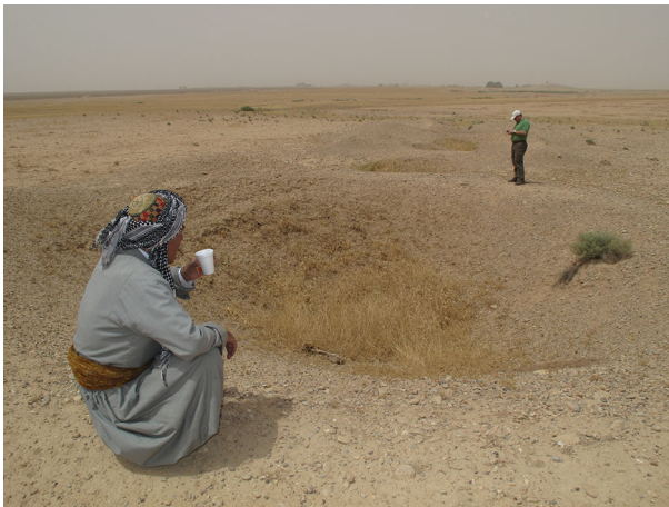
Fig. 8 Chain of wells of an abandoned qanat in Iraqi Kurdistan
