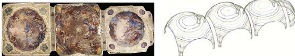
Fig. 22 Geometric survey of St. Maria church in Scaria d’Intelvi showed variations in the shapes of the three, apparently similar, vaults, that lead to the hypothesis of different construction periods. (Brumana et al. 2013)
