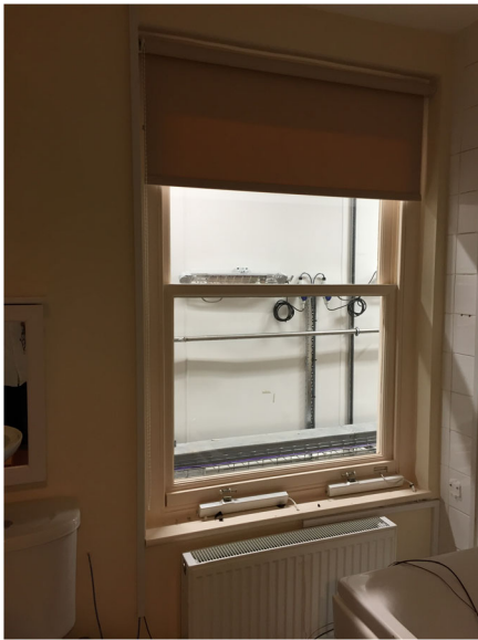
Fig. 9 Bathroom with roller blind and radiator directly beneath window
