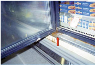
Rust indicates poor anti-condensation heating control setpoints in supermarket refrigeration cabinet [Sellers and Zazzara 2004]
