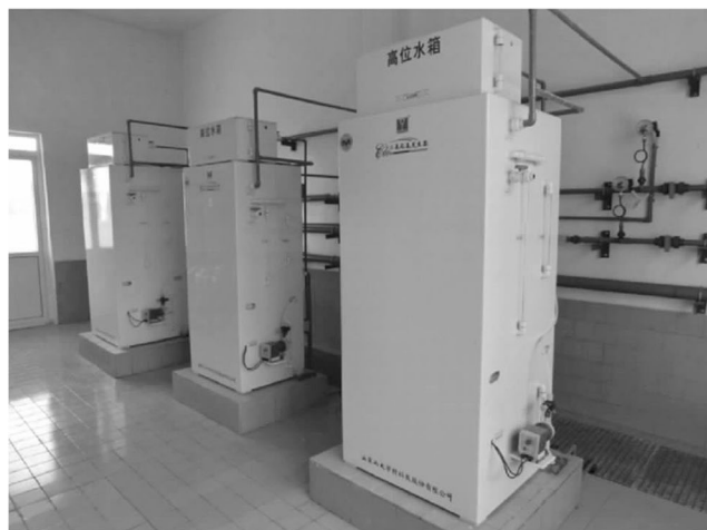
Fig. 1 A kind of chemical generator of \text{ClO}_2 gaseous in industrial system and experimental system, respectively (Deshwal and Lee 2004; Li et al. 2014)
