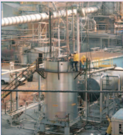
Full scale neutralizer tank test with ammonium nitrate
