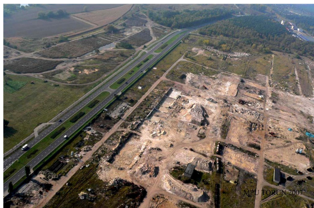
Fig. 2 Aerial view of “Polchem” after demolition ( http://archiwum.mpu-torun.pl/index.php?m=gal&id=13 )
