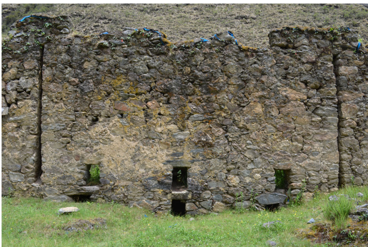
Fig. 1 A series of Inca storehouses near Cusco (Peru), with ventilation apertures visible along their lower exterior walls
