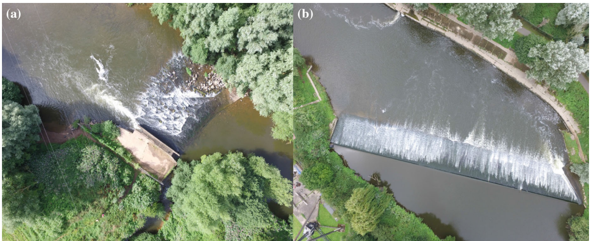
Fig. 2 Aerial images taken from a drone in 2016, of a Powick weir, located between receivers 3 and 4 in the River Teme, and b Diglis weir, located between receivers 12 and 13 in the River
