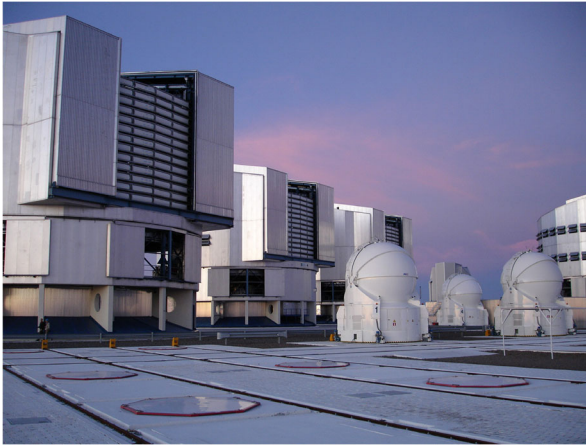
Fig. 1 The Very Large Telescope observatory features four 8.2 m unit telescopes, four 1.8 m auxiliary telescopes, and the infrastructure for performing optical interferometry. Image Credit: S. Kraus
