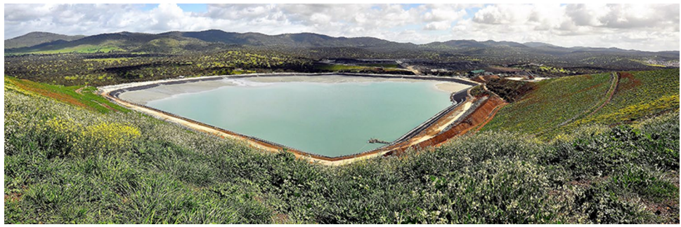
Fig. 1 A photograph of the Aguablanca nickel and copper mine tailings storage facility in Spain
