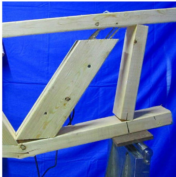
(c) Failure phenomenon
