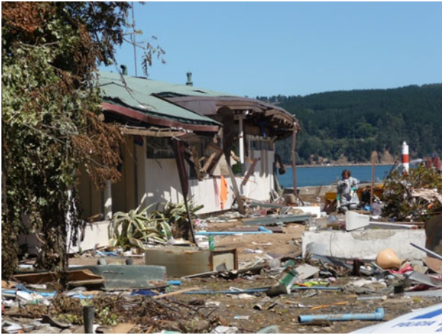
Fig. 1 Marine Station at Dichato, Chile, wrecked by tsunami in February, 2010 (photo from Dr. Camila Fernandez)
