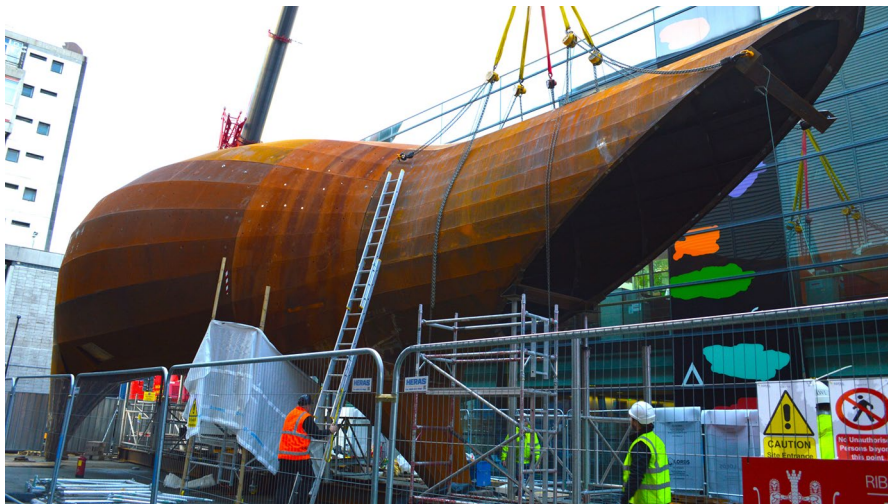
Fig. 11 Neuron pod during installation
