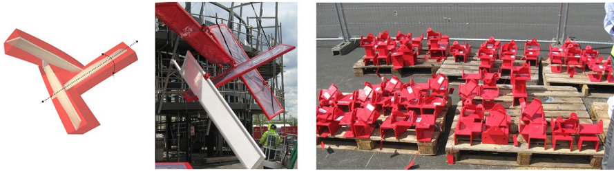
Fig. 3 Reciprocal frame, installation and custom bracket system
