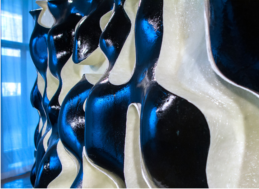
Fig. 9 The rear side of the wall reveals the thinness of the construction
