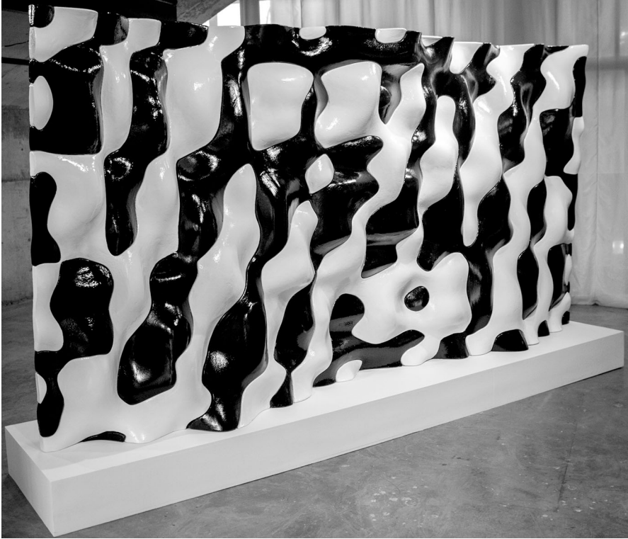
Fig. 8 Full-scale, free-standing stereotomic wall made from molded GFRP parts
