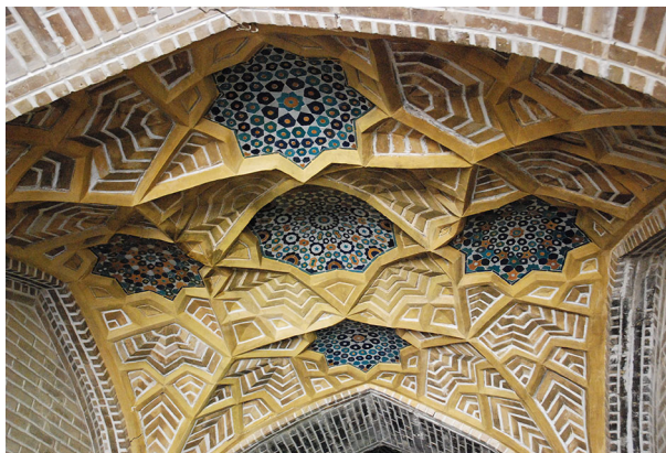
Fig. 1 Ornamented ceiling of the entrance corridor to the Kukeldash Madrasah in Bukhara, Uzbekistan. The ribbed ceiling (details in text) contains a central, two axial and two lateral mosaics delimited within eightfold star shapes
