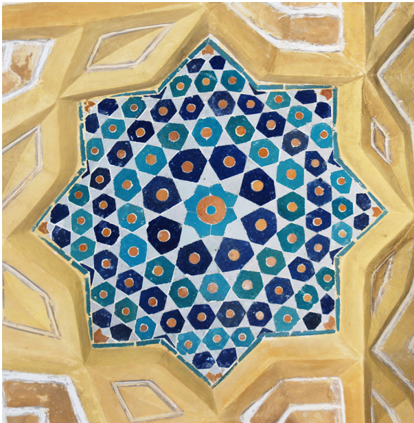
Fig. 3 The curvilinear pattern of irregularly cut hexagonal tiles from the entrance of the Kukeldash Madrasah
