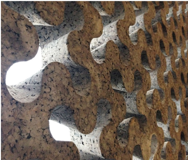
Fig. 3 The Clover Panel and the ruled surface geometry of its openings
