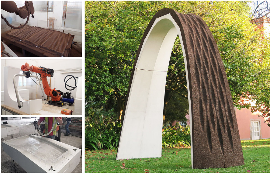
Fig. 8 The fabrication of the CorkCrete Arch ( left ) and its final installation at FAUP
