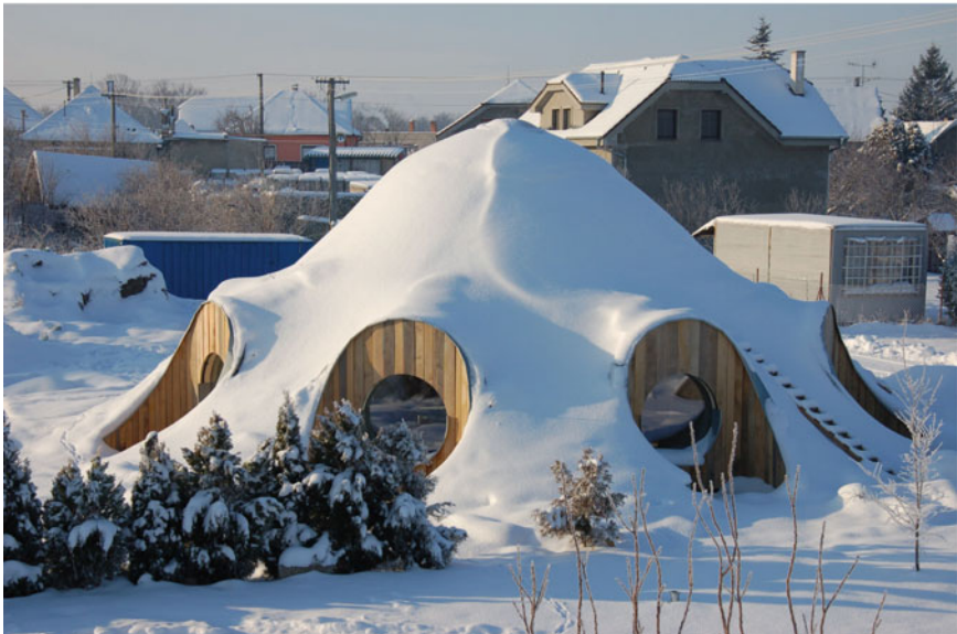
Fig. 4.21 Unique loadbearing strawbale dome. Photograph courtesy of Createrra
