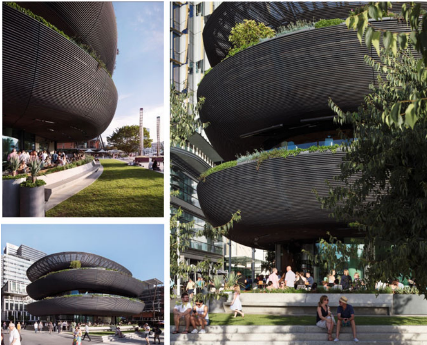
Fig. 4.17 Barangaroo house. Photograph courtesy of Rory Gardiner
