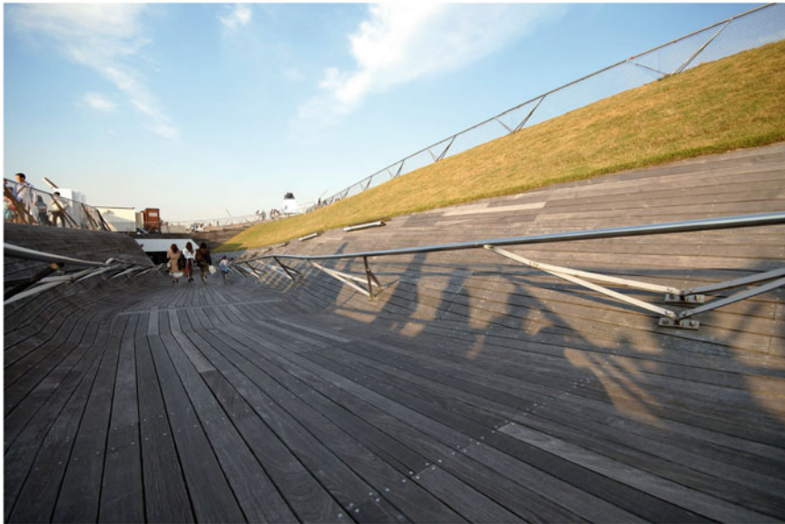
Fig. 4.14 Yokohama Ferry Terminal
