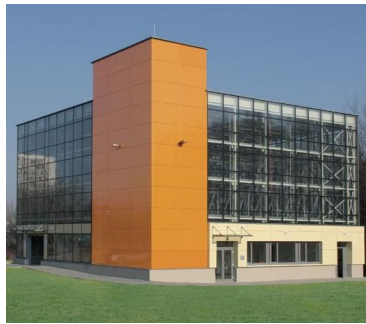
Fig. 1. A view of the Automated Transportation Center in Ostrava
