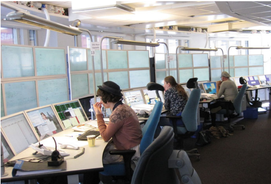
Fig. 2. The same control centre as in Fig. 3, but here re-designed for visualization using a number of large size screens at each individual workplace.
