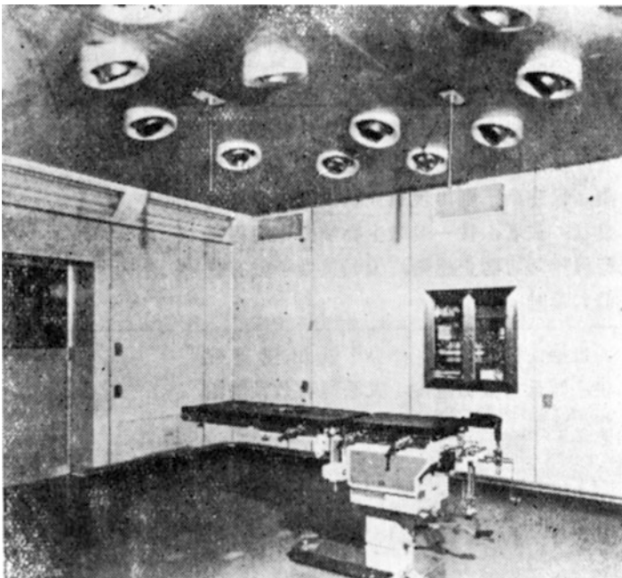
Fig. 9.22 Shadowless lamps inlaid in the ceiling
