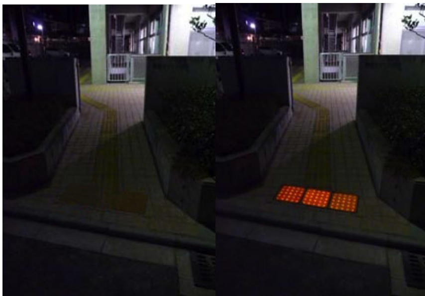
Fig. 2. Example of light-emitting textured paving block by using LED
