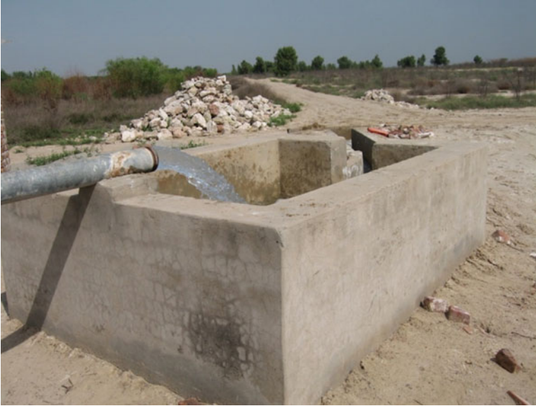
Plate 3.4 Vertical drainage through installing tube well (an example from Pakistan); the poor quality groundwater is used to irrigate salt tolerant plants at the Biosaline Research Station of NIAB, Pakka Anna near Faisalabad. Gypsum stones are also seen which are used as amendment for mitigating the high SAR and RSC (Residual sodium carbonates) levels of the water
