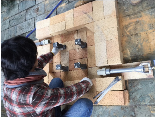
Fig. 7. Paving the pedestal of an outdoor raku kiln
