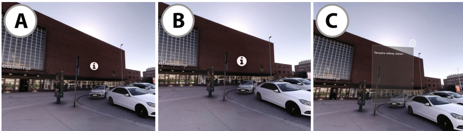
Fig. 1. Interaction with hotspots. A: A hotspot is embedded on a building. B: The user focuses the hotspot at the center of the viewport, and the hotspot starts growing to visualize dwell time. C: The hotspot is triggered, and the content is shown.
