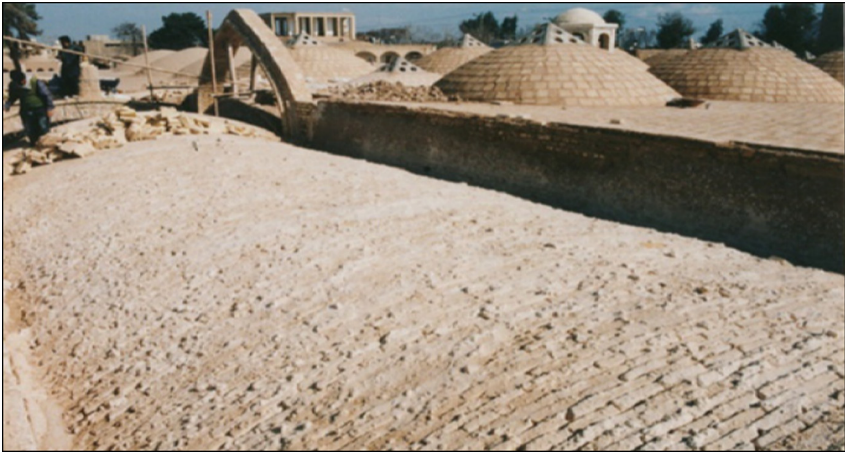
Fig. 1. External view of the case study vault
