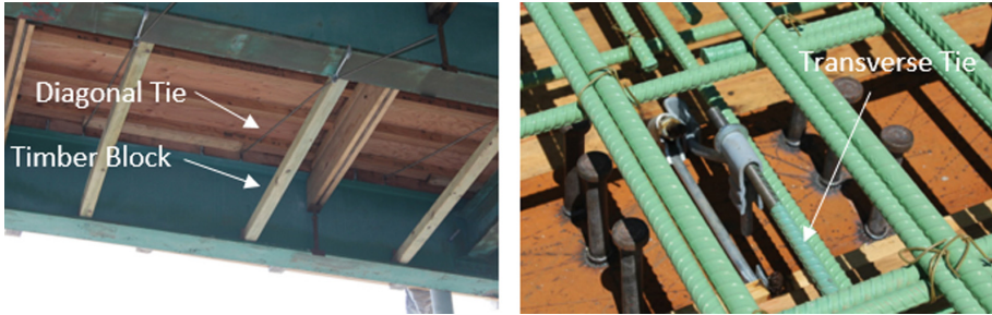
Fig. 2. Transverse and diagonal ties installed during bridge construction
