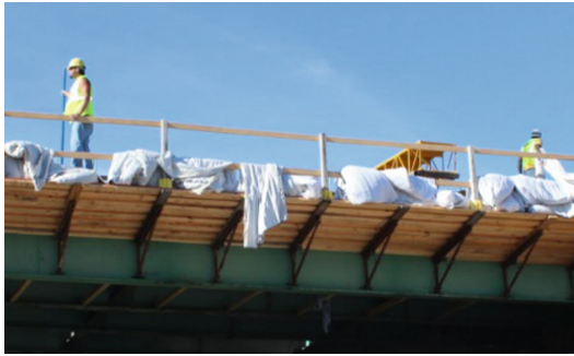
Fig. 1. Deck overhang in bridge construction
