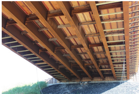
Fig. 3. Placement of timber blocks at the exterior panels of a bridge
