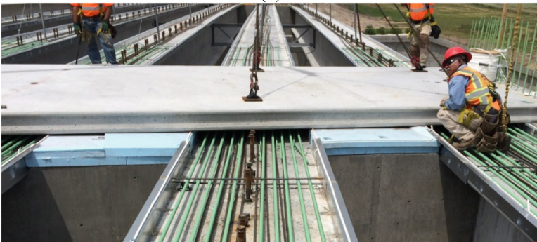
Fig. 9. Erection of precast concrete deck panels.
