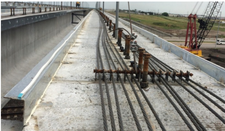
Fig. 7. Deck support system and post-tensioning strands.
