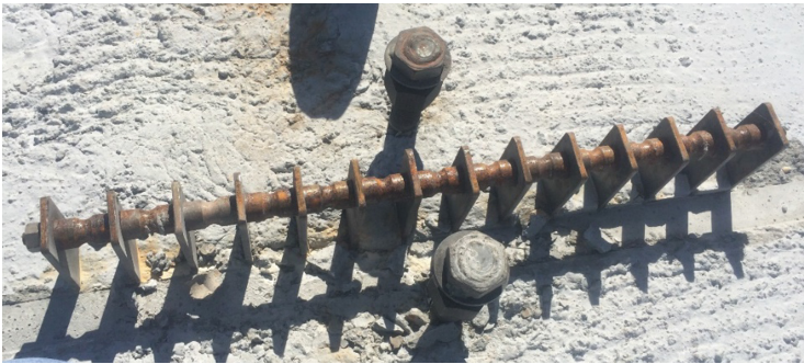
Fig. 3. Post-tensioning strand deviators
