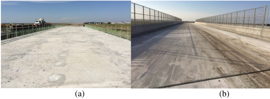
Fig. 13. Final deck surface: before grinding (a), and after grinding (b)
