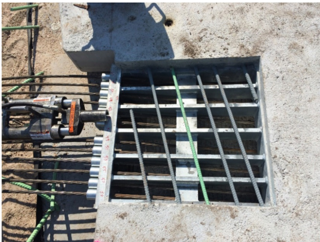
Fig. 11. Post-tensioning strands and anchor block.
