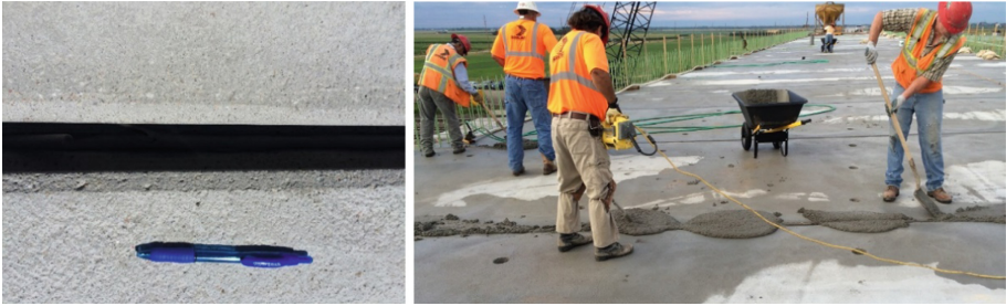
Fig. 10. Placing concrete for transverse joints.
