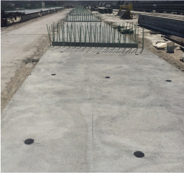
Fig. 6. Completed panels at the precast yard before shipping
