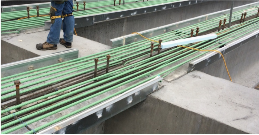
Fig. 8. Live load continuity reinforcement over intermediate support.
