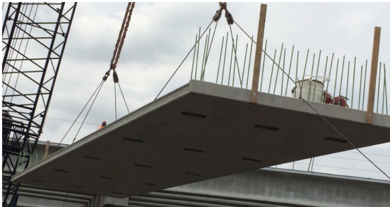
Fig. 8. Live load continuity reinforcement over intermediate support.
