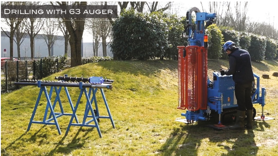
Fig. 8. In situ pressuremeter testing
