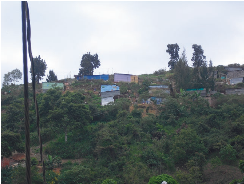
Photo 9.1 Ranchos in Casaalta 4, according to local residents built in unstable soil. Photo by the author
