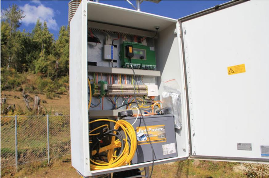
**Fig. 2.3** Rara Nepal. OTT data logger and data transmission modem in IP65 enclosure
