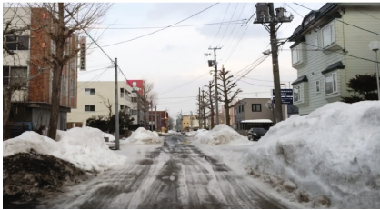
(e) sherbet road surface with potholes
