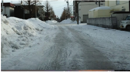
(c) frozen road surface with potholes
