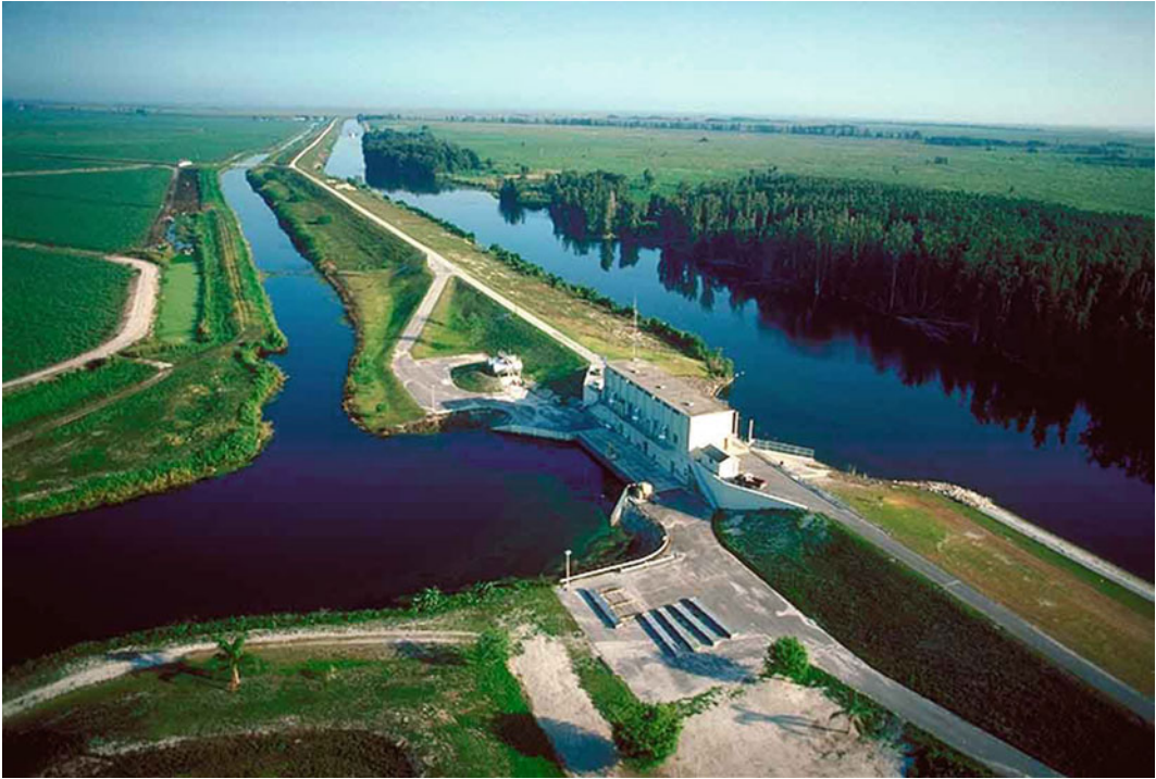
Fig. 1.11 Pump station on a drainage canal in southern Florida (South Florida Water Management District)
