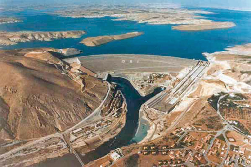
Fig. 1.2 Ataturk Dam on the Euphrates River in Turkey (DSI)
