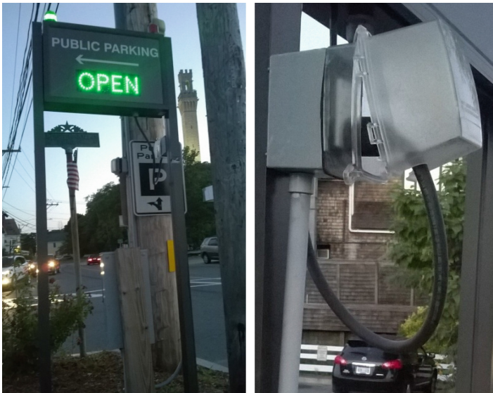
Fig. 6. In 2014, Provincetown, Mass. introduced a solution that is aimed to improve the traffic flow in this popular resort town. Unfortunately, the operator of the largest municipal parking lot has to take a 10-minute walk in order to manually switch the signal indicating the actual situation in the parking lot. That is by switching the electric cord to another outlet.
