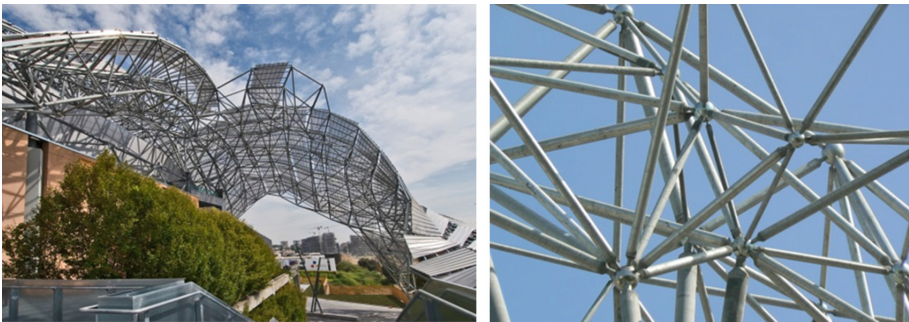
Fig. 5. “Cometa” Milano Portello Fair in Milan (arch. M. Bellini, struct. eng. M. Majowiecki)
