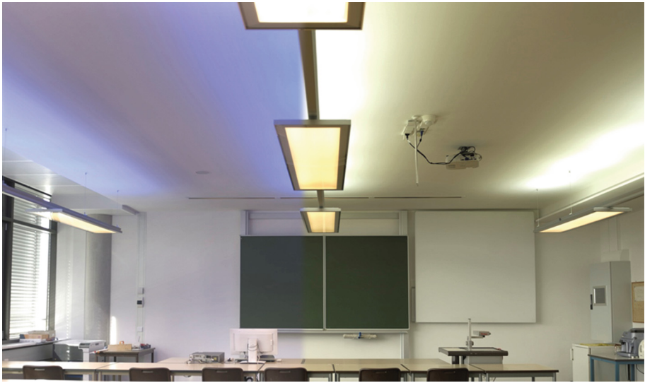
Fig. 1. Photographic picture of the Munich seminar room with the biologically effective light system, the picture consists of two different parts: left: 100 % blue LEDs and 0 % white LEDs are switched on, right: 100 % white LEDs and 0 % blue LEDs are switched on. Between these two stages, the software calculates the dynamic curve which will be shown below (see: Fig. 2)
