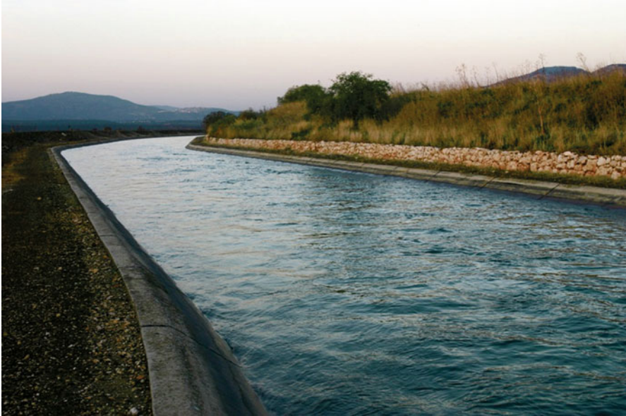
Fig. 16.3 National Water Carrier of Israel (Photo: Mekorot)
