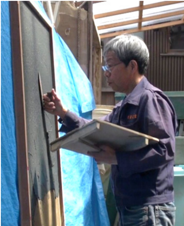
Fig. 1. Kyoto-style earthen wall process
