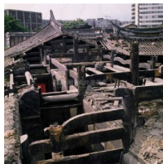
Fig. 3. The old house was in a removal proceeding
