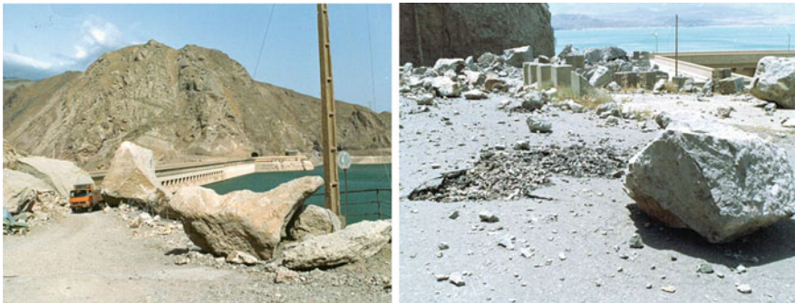
Fig. 20.6 Access roads to Sefid Rud dam site blocked by numerous rockfalls caused by the 1990 Manjil earthquake in Iran
