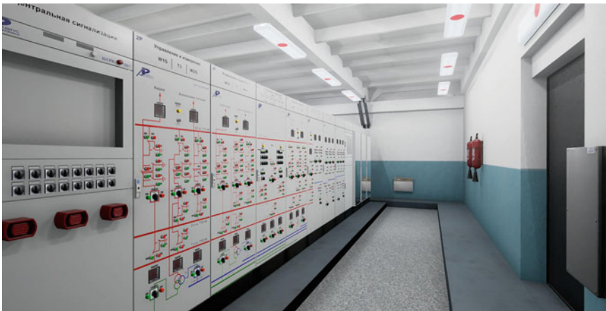
Fig. 19.8 3-D model of the main control room
