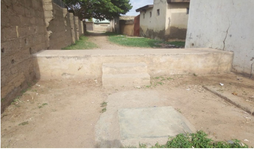
Fig. 10 Resident adaptation measures (coping strategy) to flood, to hold back and/or divert flood water away from their residence (Gwammaja)
