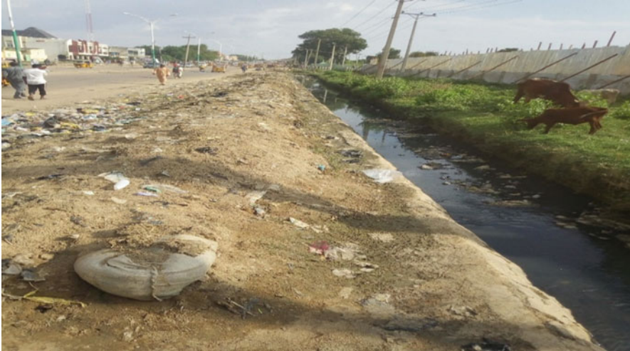
Fig. 11 De-siltation of drainages to improve free flow of storm water, but not properly evacuated which have tendency of finding its way back into the drainage
