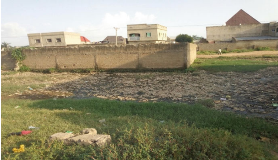
Fig. 6 Abandoned development in a low-lying area due to adverse effect of flooding in the study area (Kofar Ruwa quarters). (Source: Field Survey 2019)
