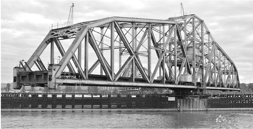
Figure 1. An open BNSF railroad swing bridge [18].
